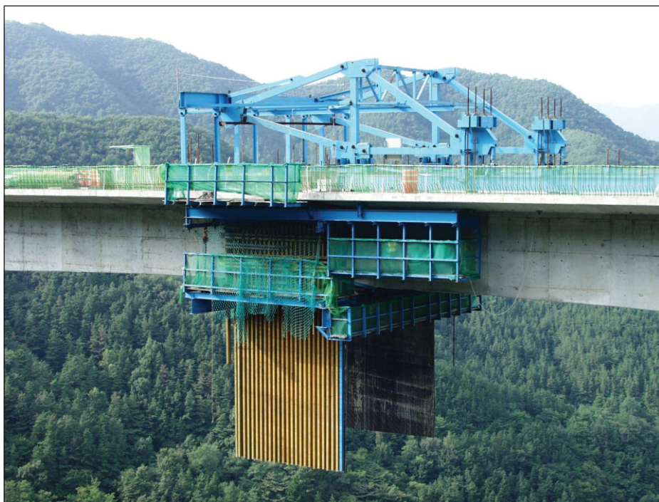
Fig. 9: Midspan closure (key segment)
