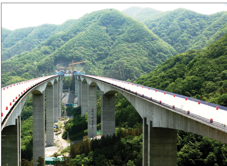
Fig. 2: Shin Chon Bridge shortly before completion
