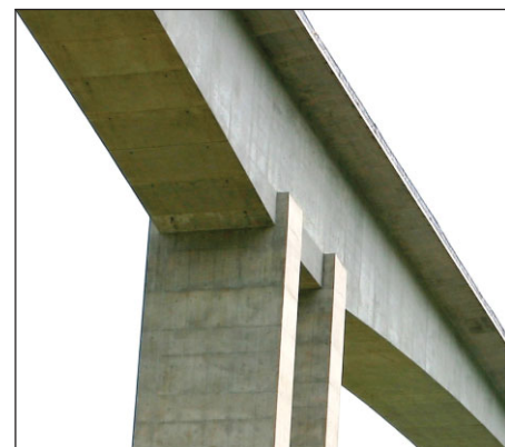
Fig. 6: Superstructure-to-pier transition
