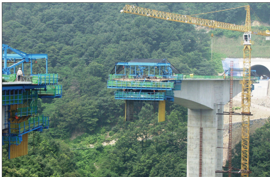
Fig. 7: Balanced cantilever construction of superstructure
